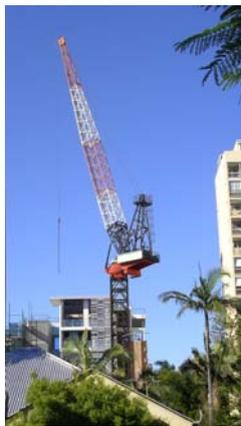
Figure 1 – Luffing tower crane
