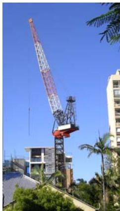
Figure 1 – Luffing tower crane
