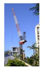
Figure 1 – Luffing tower crane
