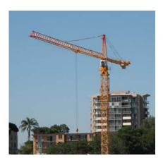
Figure 2 – Hammerhead tower crane
